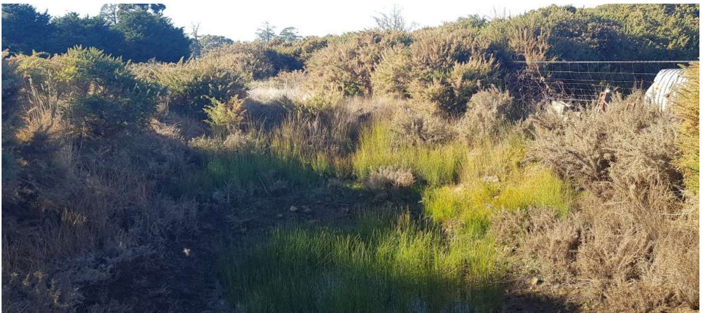
Fig.17 The existing dam is empty despite significant rainfall. The vegetation indicates it does not hold water.
